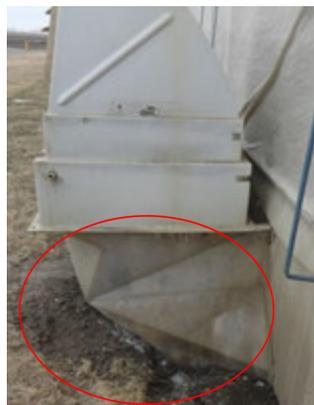
The IDNR does not accept this type of fan transition on confinement buildings.
